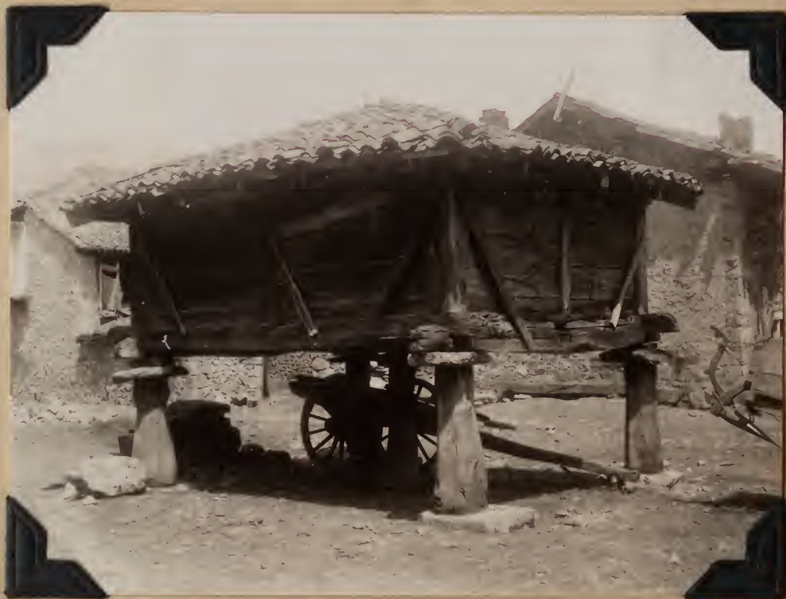
2027. Storehouse for grain in Riaño, León. Note flat stones under corners to prevent climbing rats from entering. May 18, 1930.
